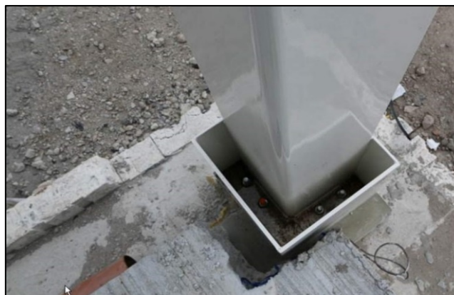
Fig. 11.9 Example of accessible base connection [137]
