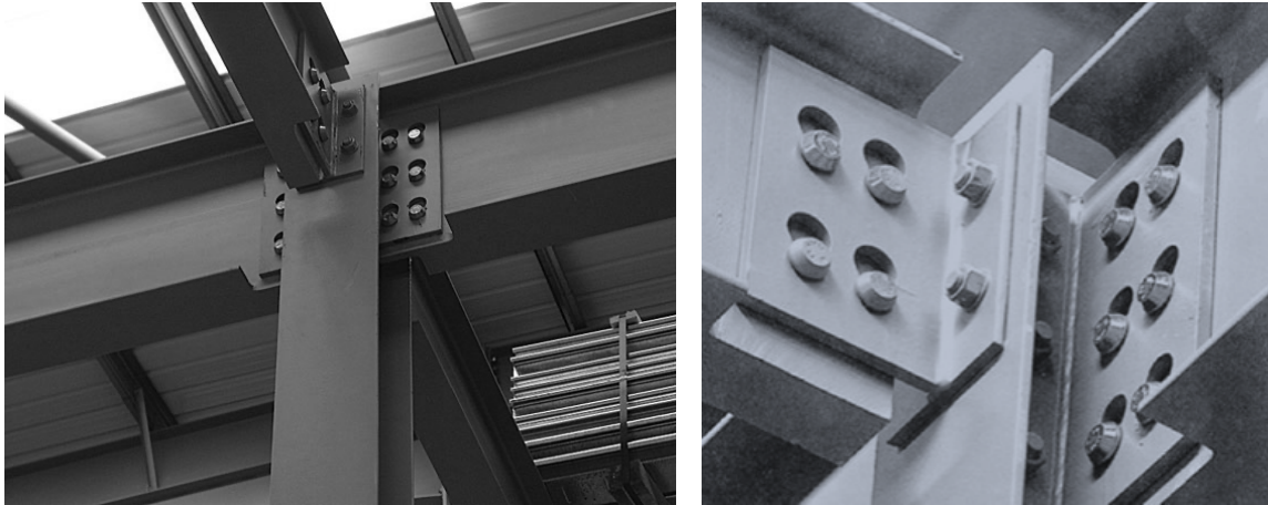
Fig. 11.16 Quicon connections [140]
