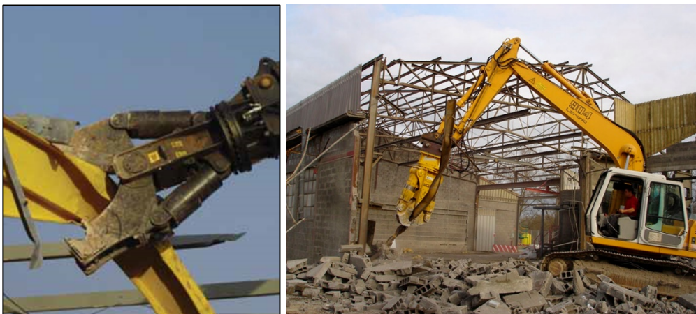
Fig. 7.8 Steel shear attachment pulling-down and shearing a steel structure
