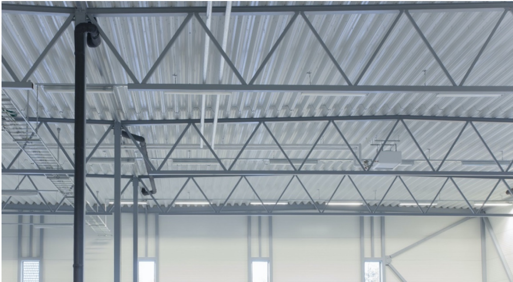
Fig. 11.23 Example of roof system with deep decking [138]
